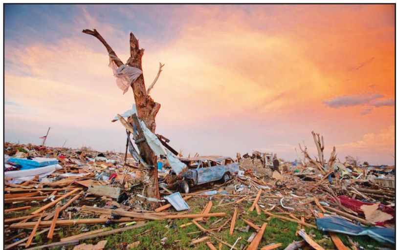
The Moore area was struck by an EF5 tornado.
