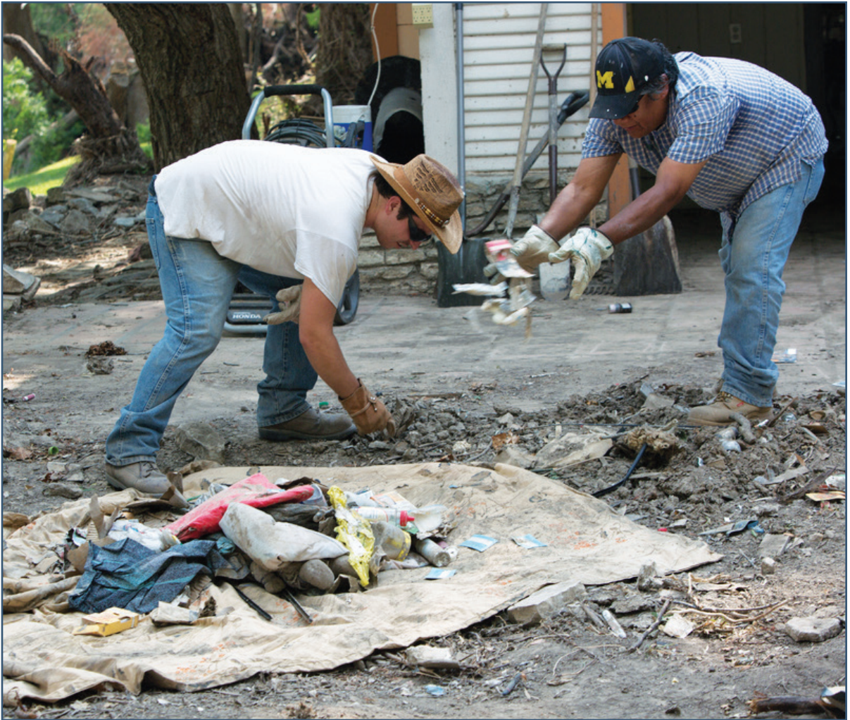
Rebuilding after flooding in Texas
