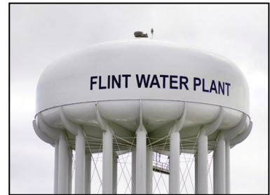
Figure 8: Flint Water Plant
